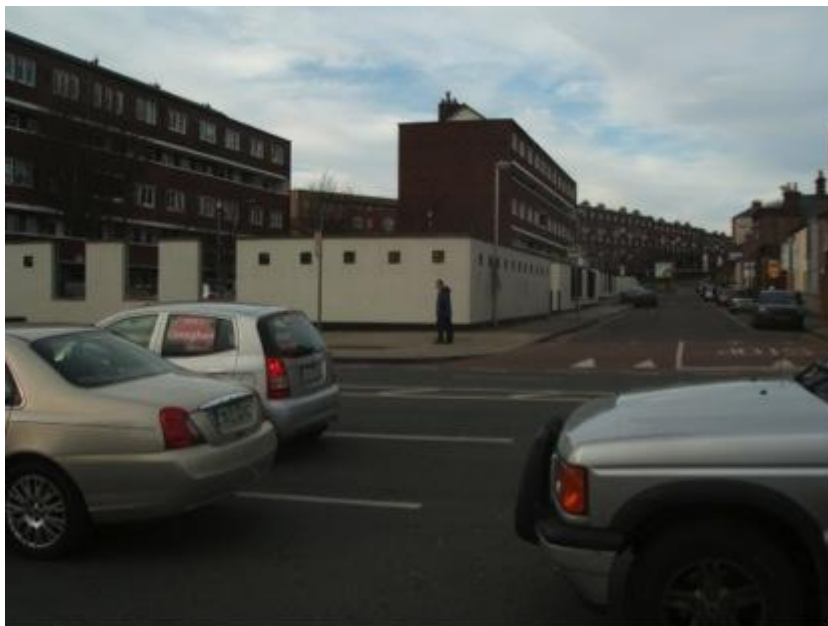
Public housing areas surrounding Smithfield
