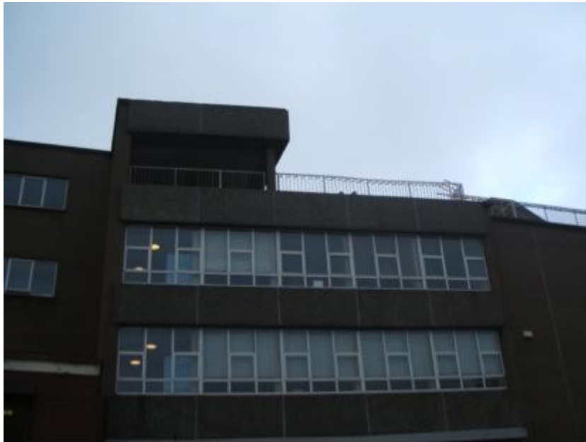
A primary school in Smithfield. The play area is on the school roof
