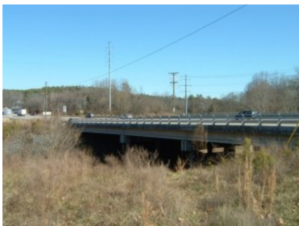
The James Taylor Bridge over Morgan Creek in his native city of Chapel Hill, North Carolina
