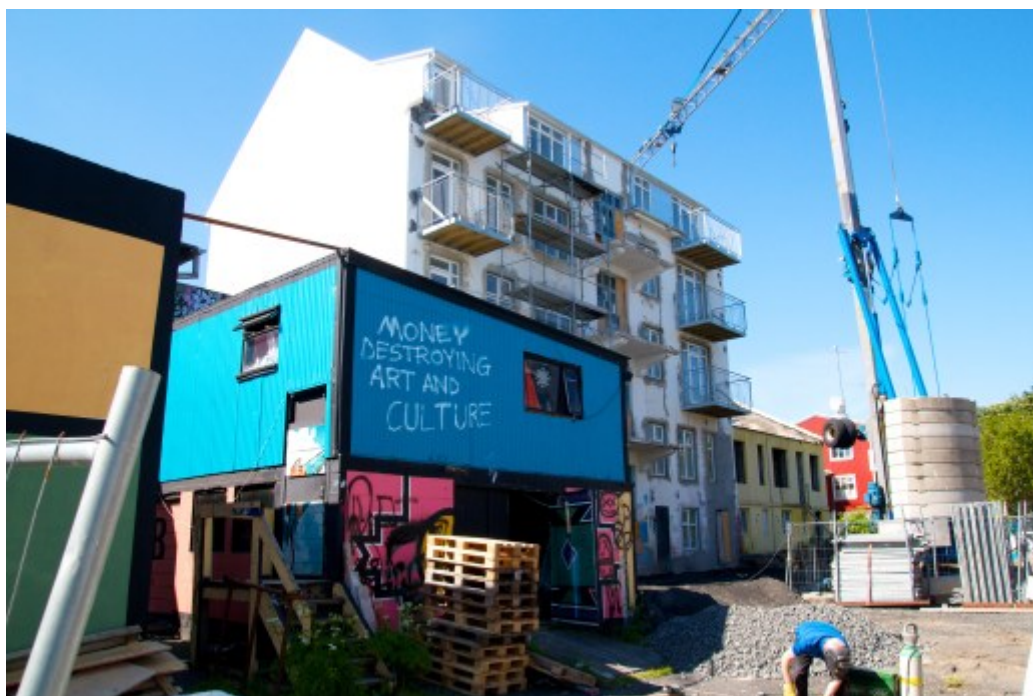
Construction in Reykjavik. Image by Patrick Rasenberg @Flickr CC BY-NC.
